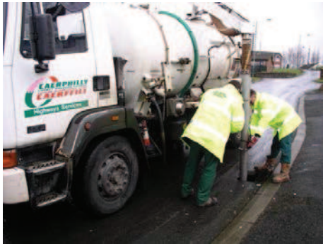
A Gully-emptier Lorry in action – cleaning a gully and jetting a manhole
