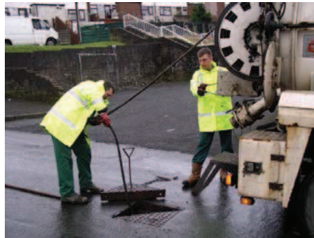
A Gully-emptier Lorry in action – cleaning a gully and jetting a manhole
