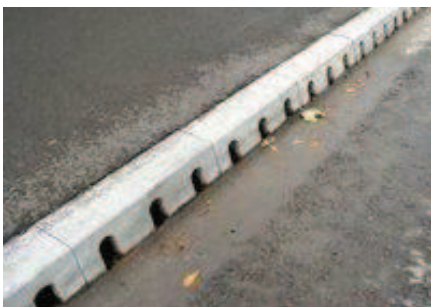
Typical Kerb Drains
